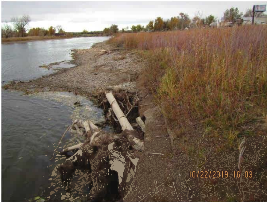
FIGURE A.5.4. Site 2 & 3 - Wyoming Blvd, standing at downstream end of toe wood 2, looking downstream.
