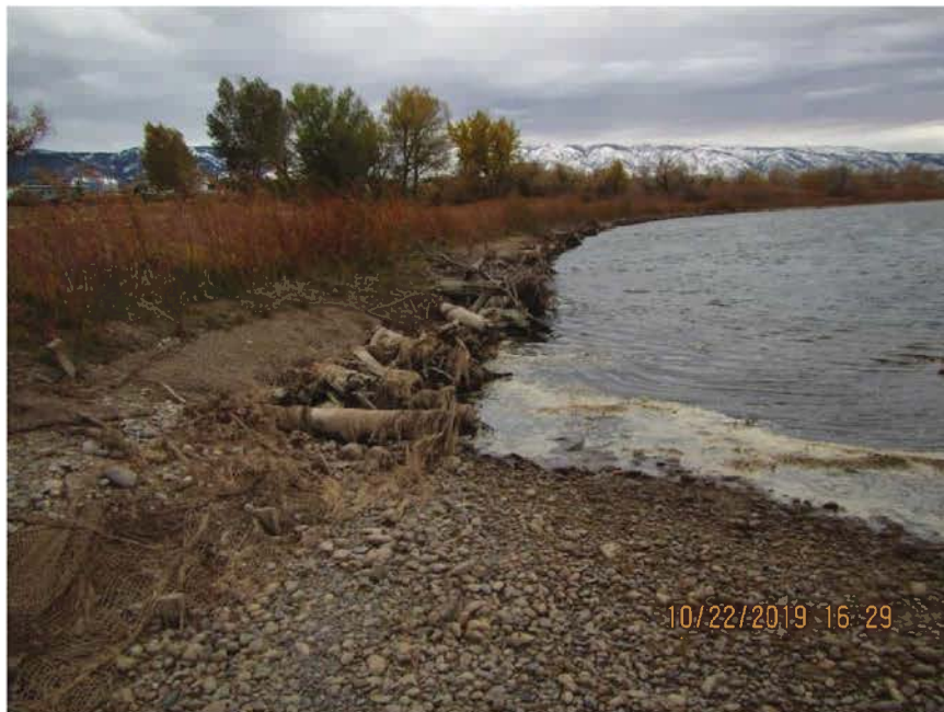
FIGURE A.5.2. Site 2 & 3 - Wyoming Blvd, standing at downstream end of toe wood 1, looking upstream. Willows have established well above the structure, contributing to long-term bank stability.
