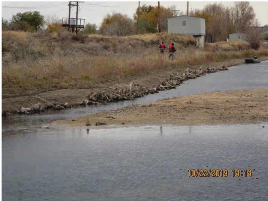
FIGURE A.5.10. Site 2 & 3 - Wyoming Blvd, standing in-stream, near upstream end of toe wood 5, looking downstream at lower half of toe wood 5.
