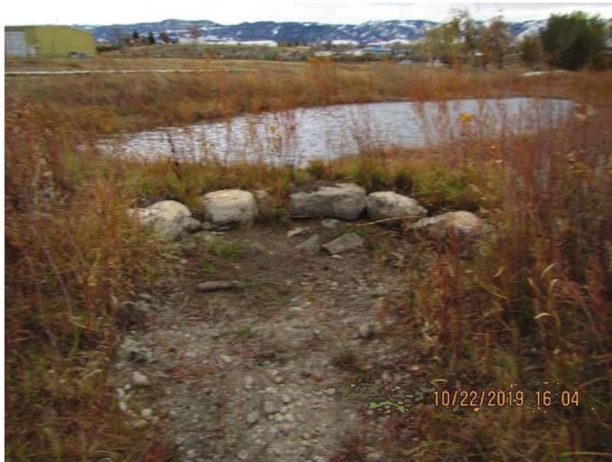
FIGURE A.5.20. Site 2 & 3 - Wyoming Blvd, at upstream set of wetland cross vanes, looking at cross vane 37.
