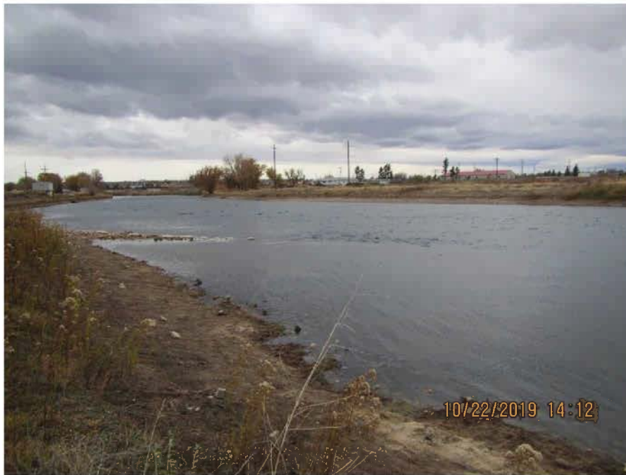
FIGURE A.5.16. Site 2 & 3 - Wyoming Blvd, standing upstream of rock vane 5 on river left, looking downstream, in at rock vane 5.
