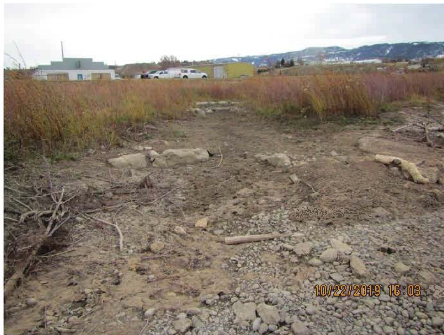
FIGURE A.5.22. Site 2 & 3 - Wyoming Blvd, at upstream set of wetland cross vanes, looking at cross vanes 39A (middle) and 39B (closest). Cross vane 38 is also visible (furthest).
